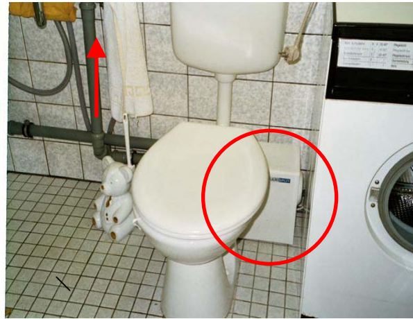
Fig. 6: Example of a pump with chopping unit
