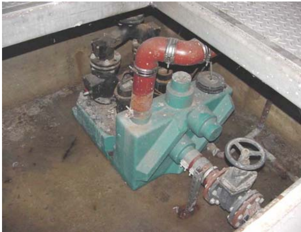
Fig. 5 Example of a central pump station
