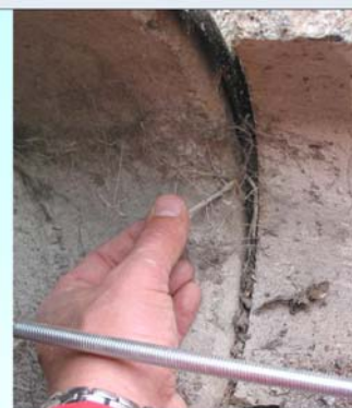
Dismantling joints Concrete "B"
