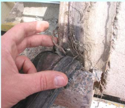
Dismantling joints Concrete "B"
