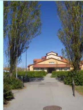
Aspen/Espen planted 1947 caused root intrusion to a new PVC-pipe constructed 2000
