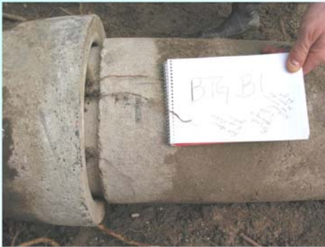
Dismantling joints Concrete "B"
