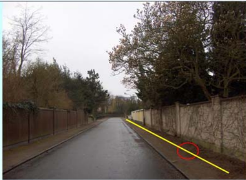
Private tree caused root damage to a public pipe after 5 years
