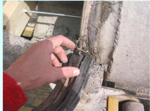
Dismantling joints Concrete "B"
